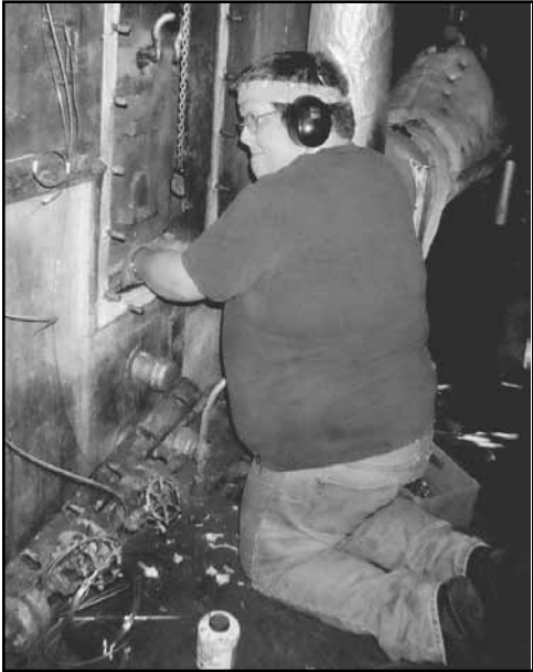
SS KAUI Wiper Theron Skewis, #3667, assisting with engine room repairs.
